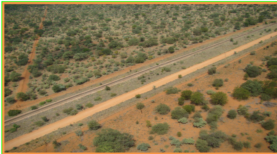
Plate 5: View of proposed powerline route running next to the existing railway line.
